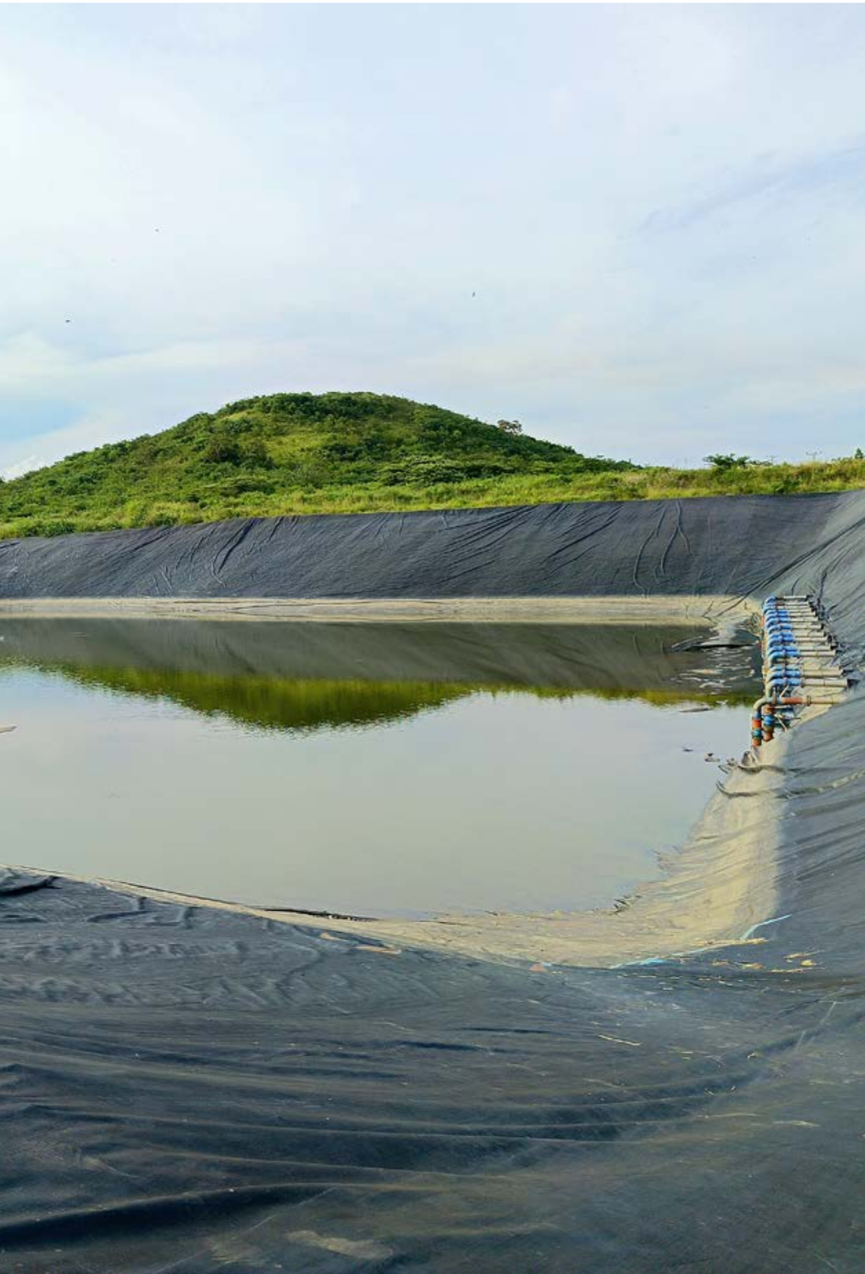
A water reservoir at one of the UDB sponsored projects.
